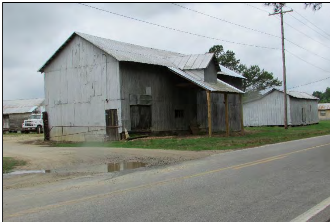
Figure 20. O.J. Smith Cotton Gin, front (north) and east elevations, looking southwest
