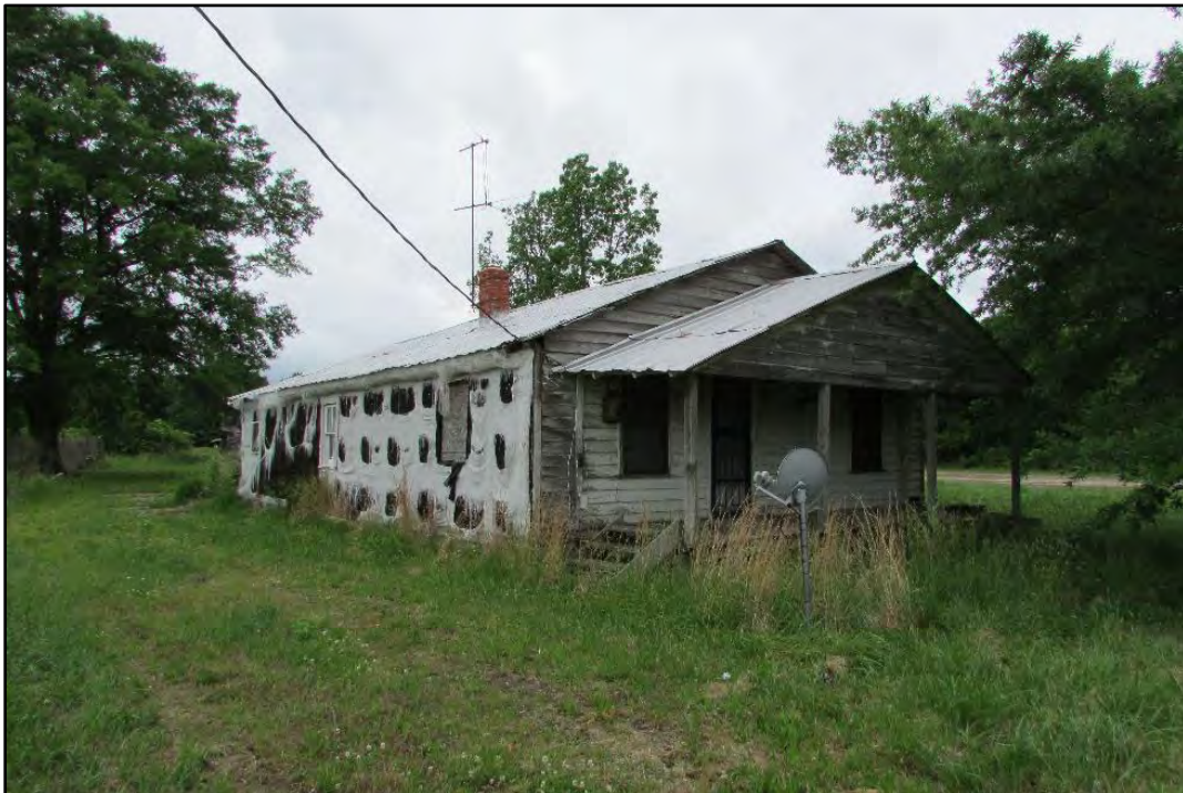
Figure 47. 8101 Swift Creek School Road (#18 on site plan), looking southwest.
