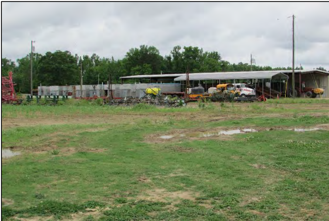
Figure 39. Pole barn and carport (#10 on site plan), looking northwest.
