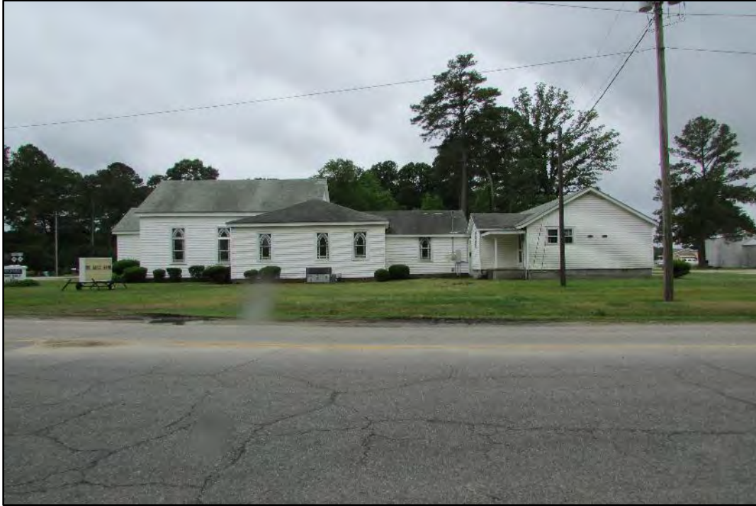
Figure 12. Hickory Baptist Church, north elevation, looking south.
