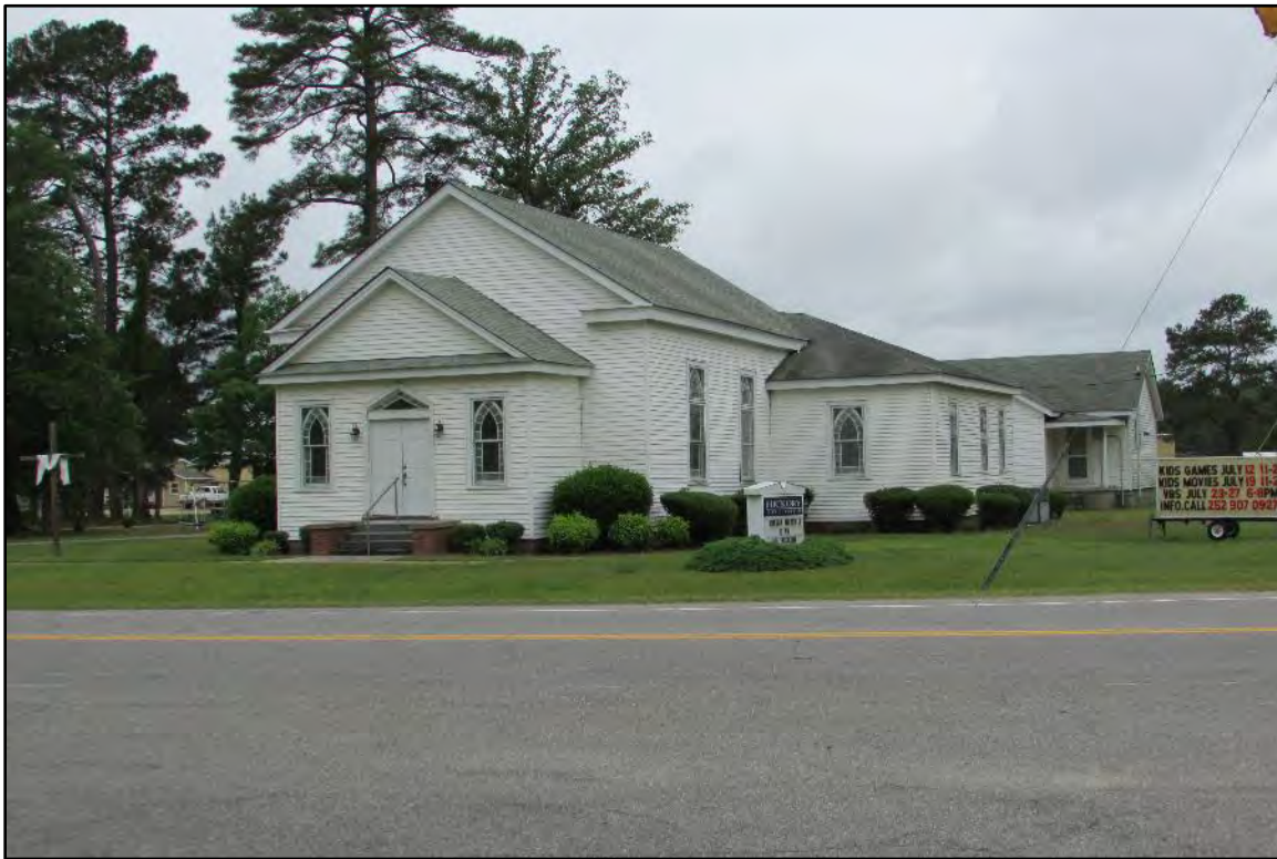
Figure 4. Hickory Baptist Church, front (east) elevation.
