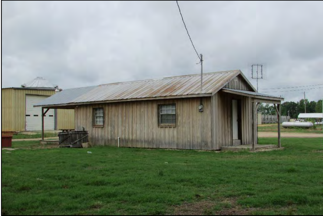
Figure 35. Office 2 (#6 on site plan), east and north elevations, looking southwest.
