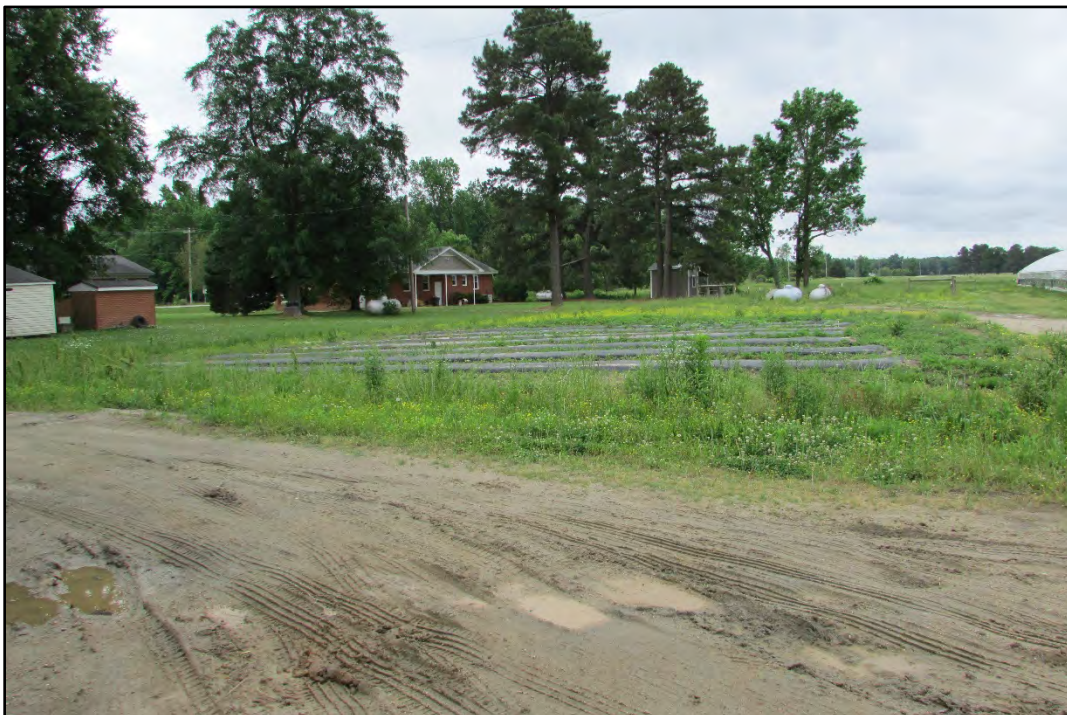
Figure 54. Looking east to the rear elevation of 12612 NC 48, which is on the same parcel.
