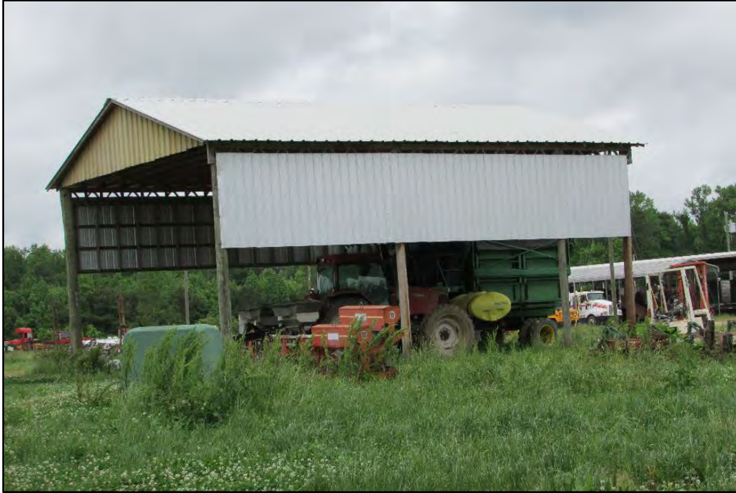
Figure 42. Pole barn (#13 on site plan), looking northwest.
