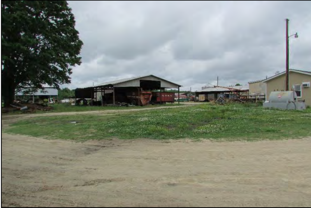
Figure 40. Pole barn (#11 on site plan), looking northwest.
