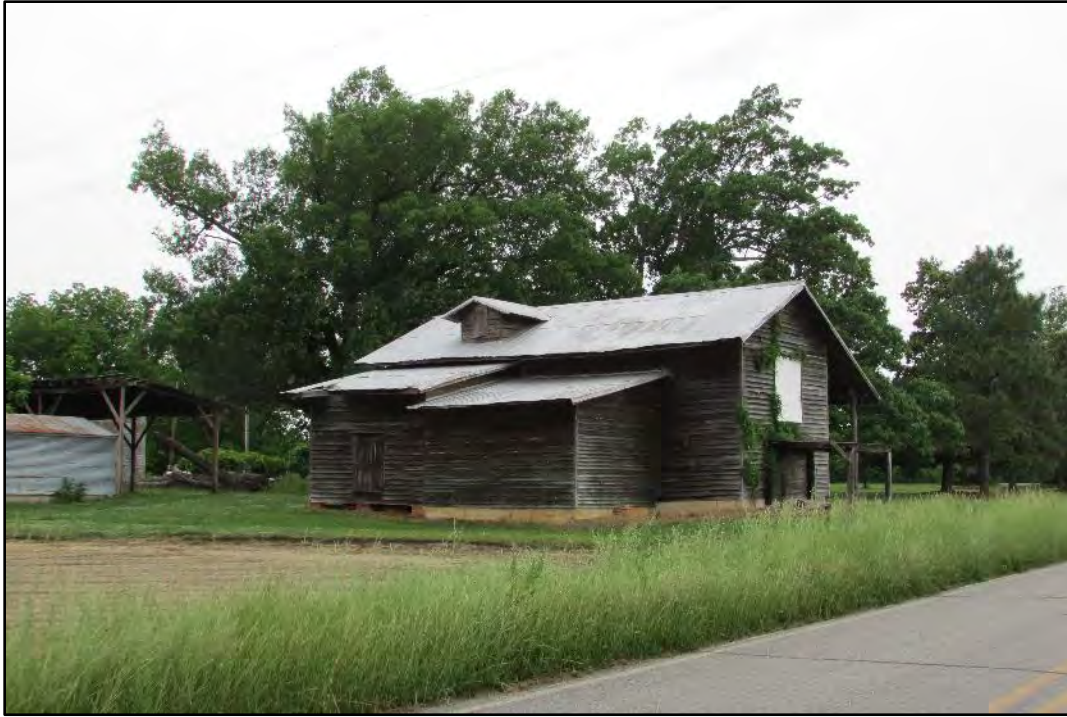
Figure 49. Davenport Cotton Gin, dating from the 1930s, south and east elevations.
