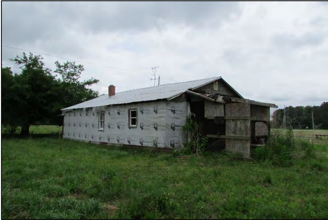
Figure 66. Smith Tenant House, 8101 Swift Creek School Road, looking northeast.
