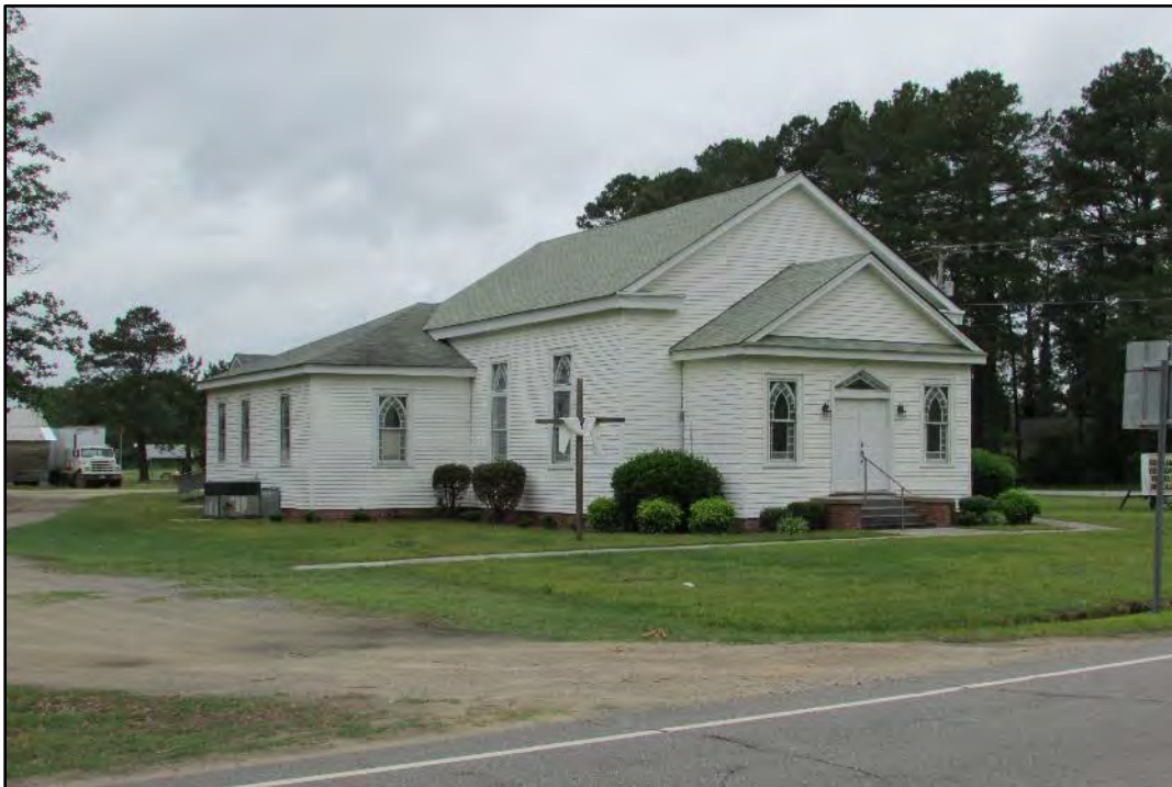
Figure 11. Hickory Baptist Church, front (east) and south elevations, looking northwest.
