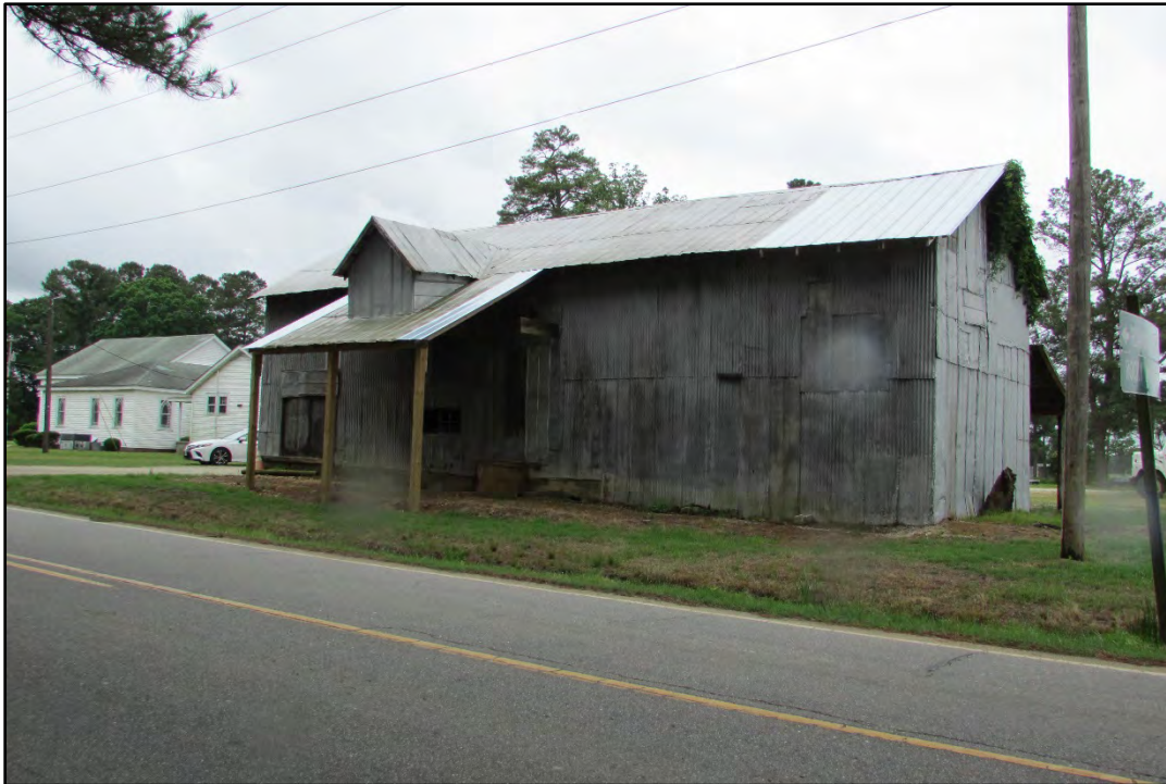
Figure 27. O.J. Smith Cotton Gin, front (north) and west elevations, looking southeast.
