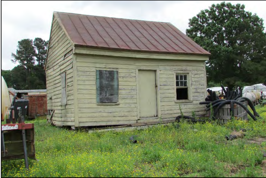
Figure 43. House (#14 on site plan), looking southeast.
