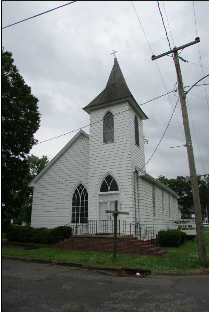
Figure 19. Whitakers Baptist Church (NS546), 105 West Pittman Street, looking southeast.
