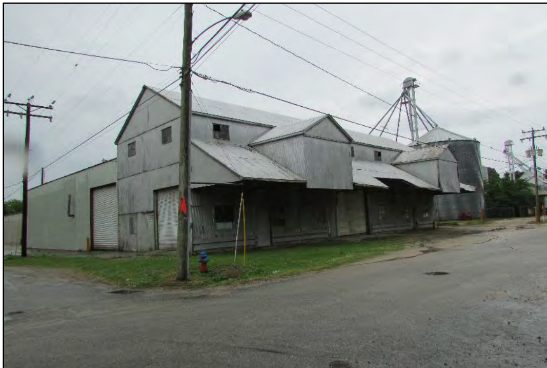
Figure 48. Cotton Gin of the Battleboro Gin & Grain Company, built after World War II, south and west elevations.
