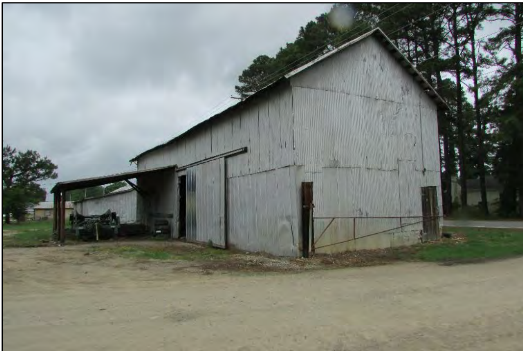
Figure 29. O.J. Smith Cotton Gin, south and east elevations, looking northwest.
