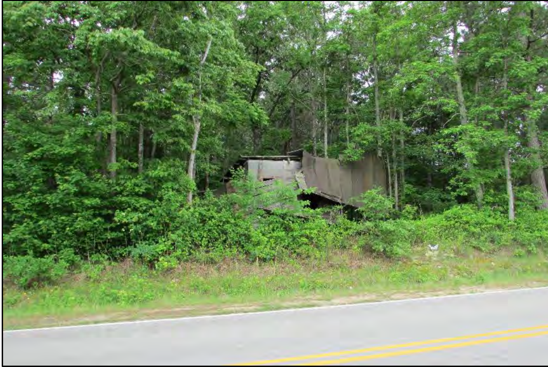
Figure 50. Cousins Cotton Gin, constructed in 1919, north elevation.
