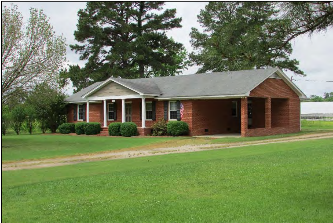
Figure 45. 12612 NC 48 (#16 on site plan), looking southwest.
