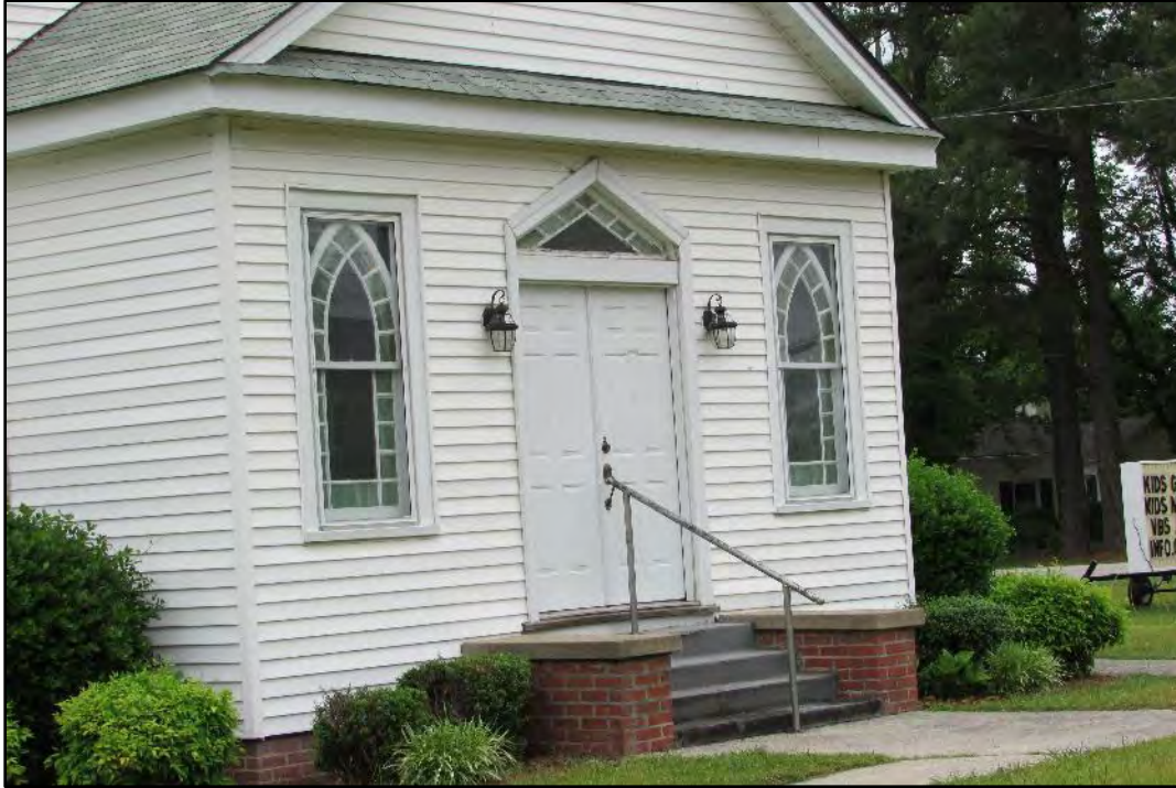
Figure 14. Hickory Baptist Church, detail of east entrance, looking northwest.
