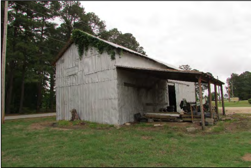
Figure 28. O.J. Smith Cotton Gin, west and south elevations, looking northeast.
