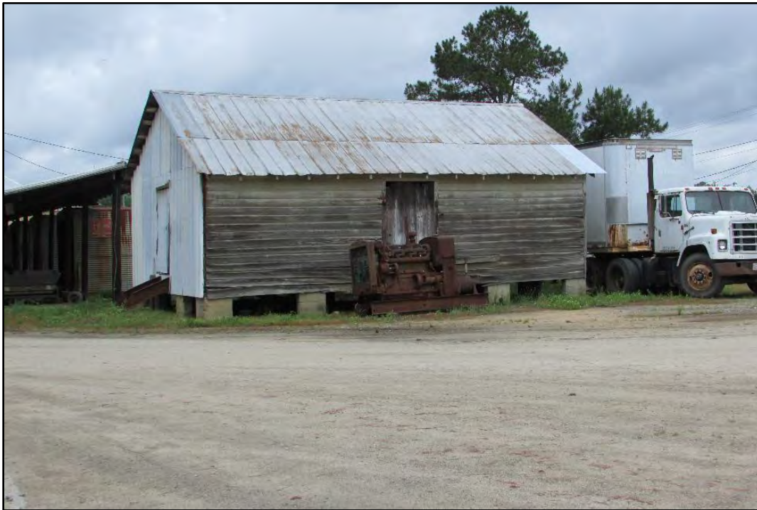
Figure 33. Warehouse (#4 on site plan), east and south elevations, looking west.
