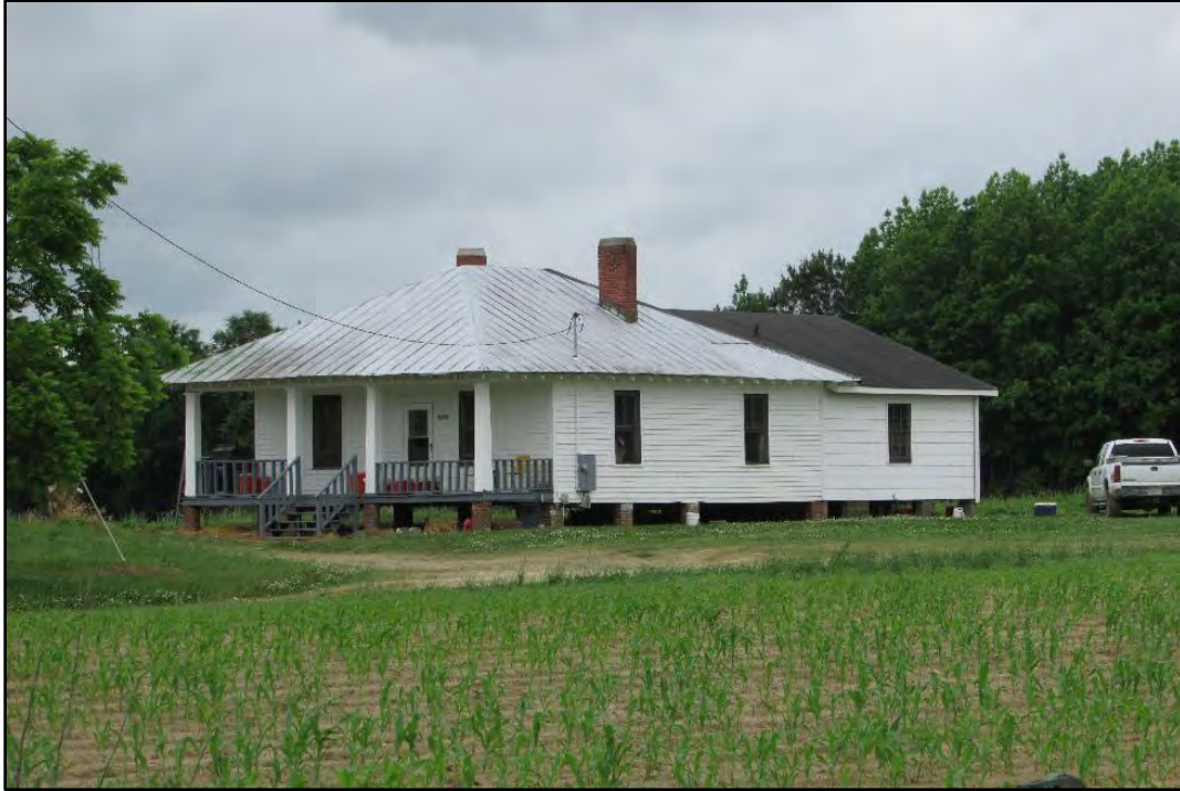
Figure 46. 12644 NC 48 (#17 on site plan), looking southwest.
