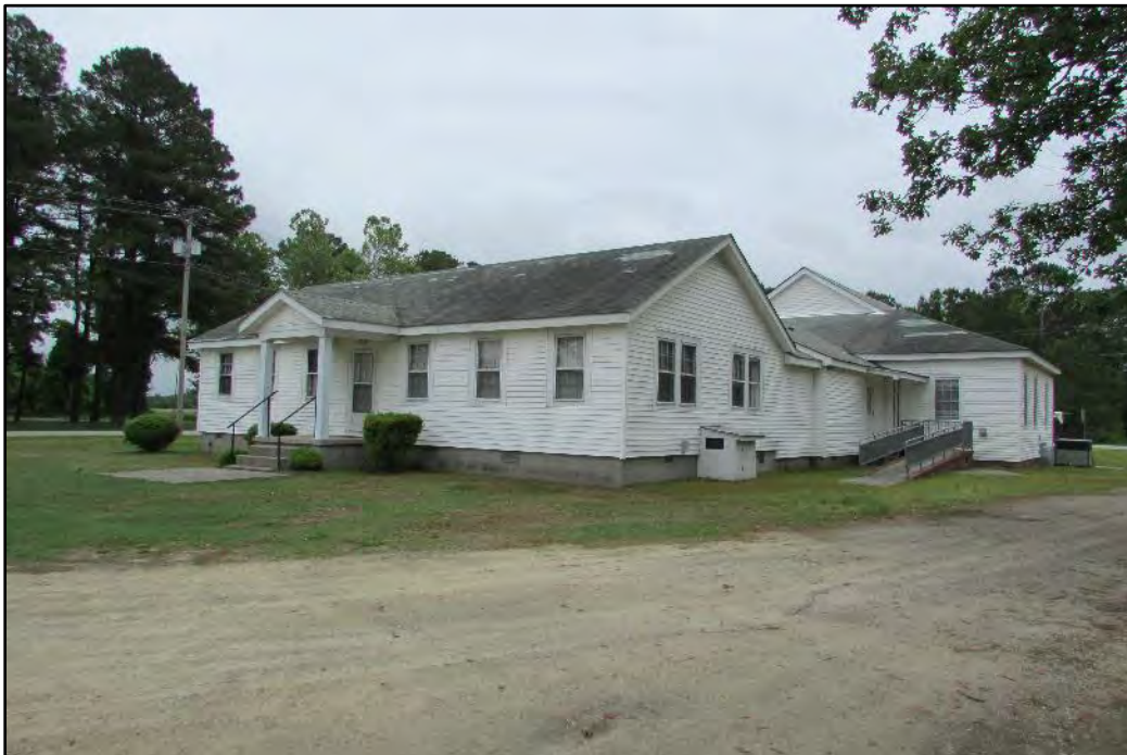
Figure 13. Hickory Baptist Church, rear (west) and south elevations, looking northeast.
