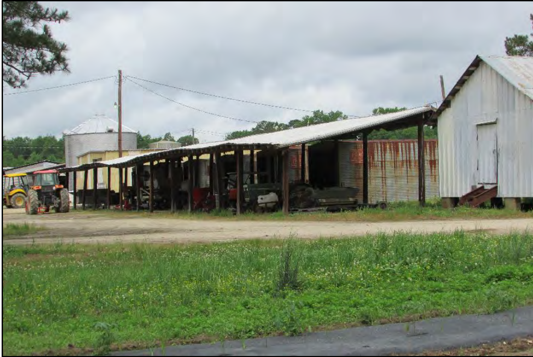
Figure 37. Pole Barn (#8 on site plan), looking west.
