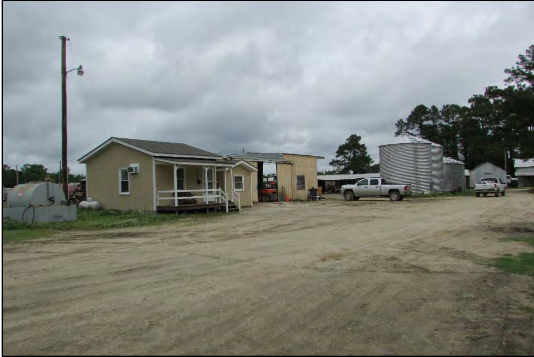
Figure 34. Office 1 and equipment shed (#5 on site plan), east and south elevations, looking northwest.
